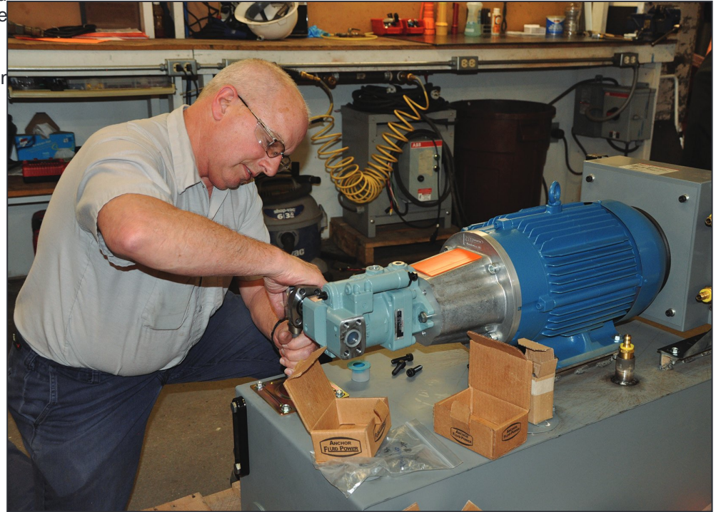
Eldon Hansen works on a Hydraulic Power Unit.
